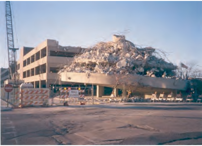
Figure 5. Deck demolition, Des Plaines, Illinois.
